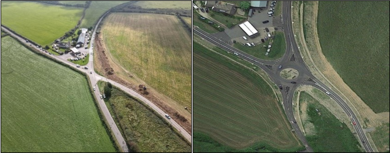
Figure 25: Lynton Cross safety improvements, with crossroads upgraded to a roundabout
